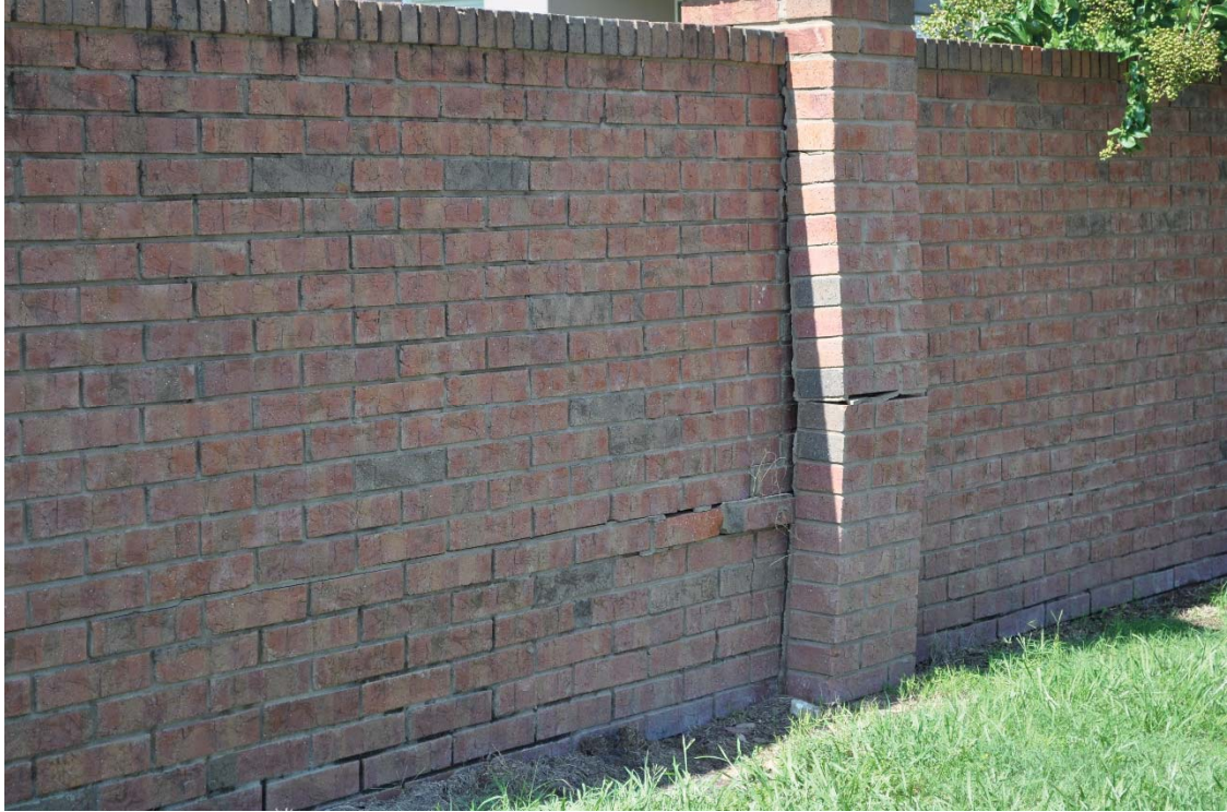
Photo B: Wall Buckling
